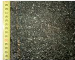
d) Very Thin Asphalt Surfacing noted "VTAC"
